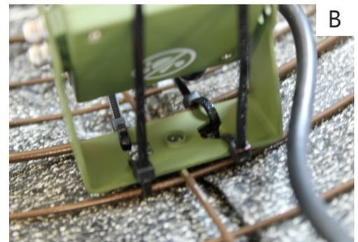
**Step 3:** Line the bracket up with the vertical pole and thread the four cable ties around the horizontal poles and through the two holes on the bracket "not the centre hole". Make sure this is secure in place as it will be flipped upside down and will fall forward. Please refer to image "B".
